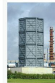
全封闭式地面火炬 Totally enclosed ground flare
