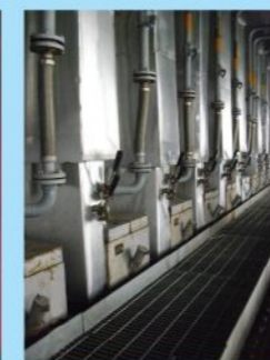
高温制氢燃烧器 High temperature hydrogen generation burner
