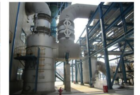
吉林石化140万吨/年催化 低压降水封罐使用现场 J.1.4 million ton/year low pressure drop water sealed tank site application in Jilin Petrochemical
